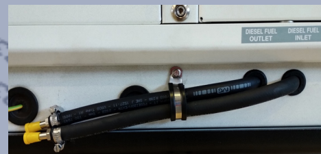
INPUT/OUTPUT FUEL PIPE
