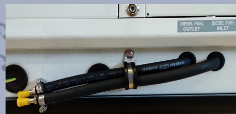
INPUT/OUTPUT FUEL PIPE
