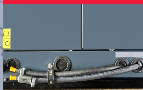
INPUT/OUTPUT FUEL PIPE
